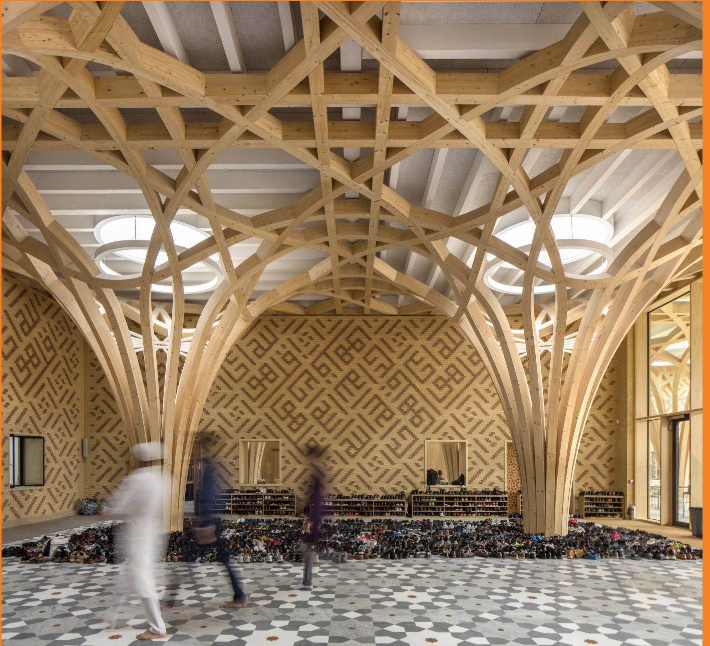
The columns are remarkably successful, bringing a grand, celebratory yet warm and welcoming sense to the internal spaces
